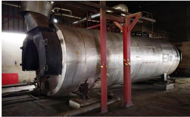
Figure 3: Furnace Oil Boiler
